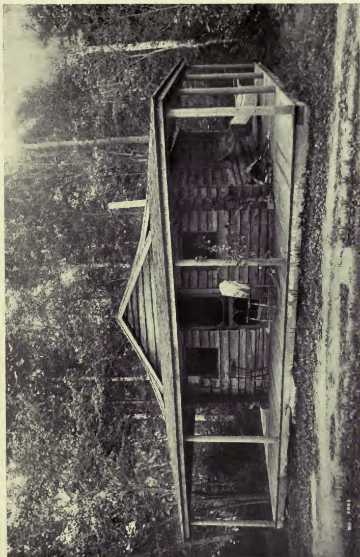
If the Roof is Very Flat in Regions of Heavy Snowfall, the Supporting Beams Should be Well Braced and of Stout Timbers.
