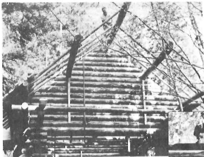
Above: Skyline Carriage which I used to put logs up on a steep, forested building site.
