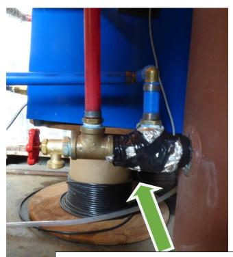
The geysers temperature probe was installed on the inlet and insulated for accuracy. It tells the geyser when to turn on and off.
