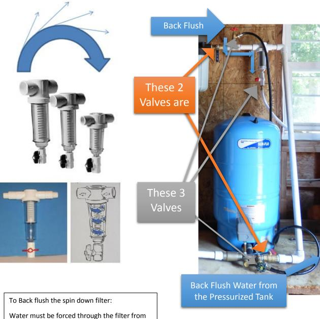
the outlet side, and out the bottom valve
