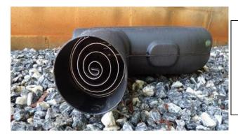
This model features a rodent guard built in, but they can also be added at the end of an overflow pipe, or where needed. A large variety are available.
